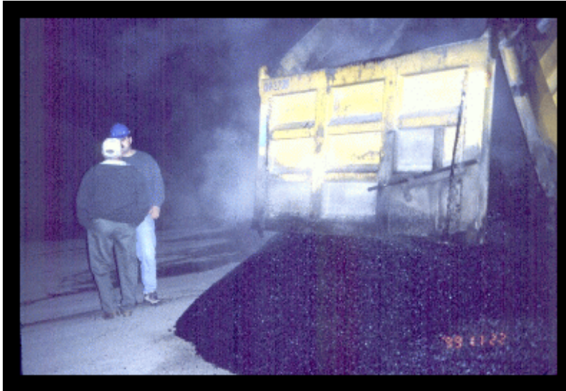
Newly manufactured recycled asphalt shingle (RAS) cold patch at Pike Industries, Williston, Vermont
