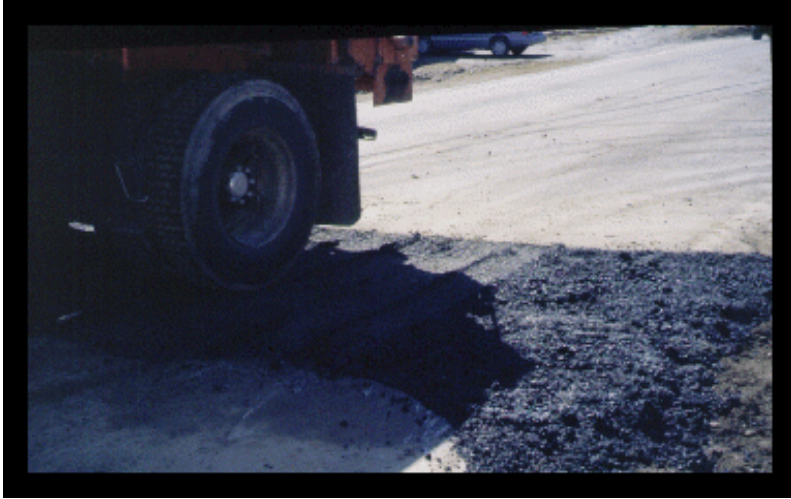
Culvert repair, VT 109, Waterville. Compacting RAS cold patch with dump truck.
