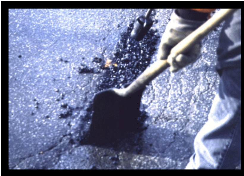
Pothole filling with cold patch, VT 14, South Barre.
