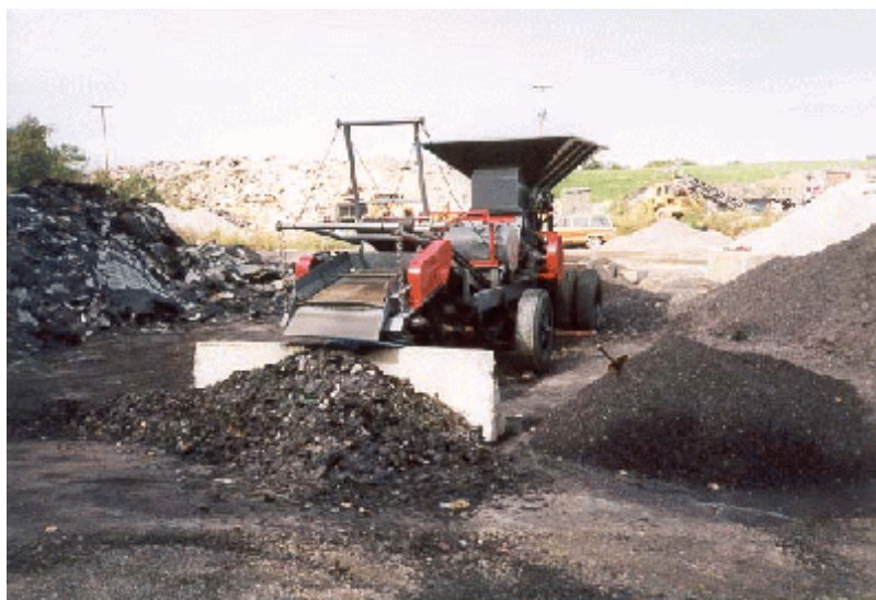
A Marcellino shingle processing equipment, South Burlington.
