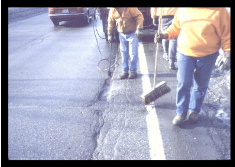
Drying potholes prior to cold patching. VT 14, South Barre
