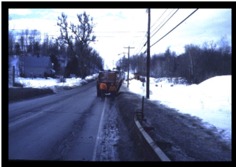
VTrans trial location for RAS cold patch, VT 14, South Barre, VT
